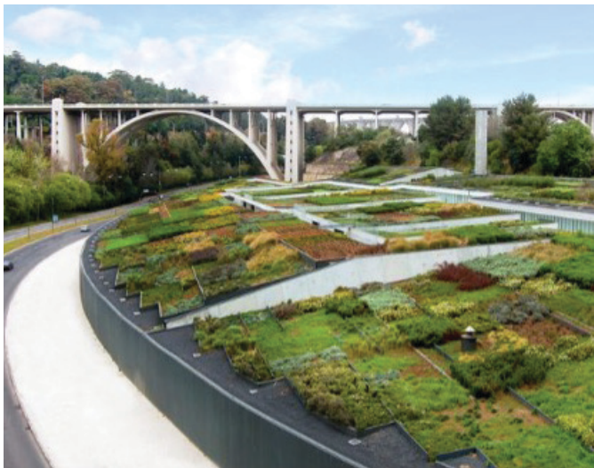
Figure 8. The Alcântara Wastewater Treatment Plant. Source: Argex AS.
