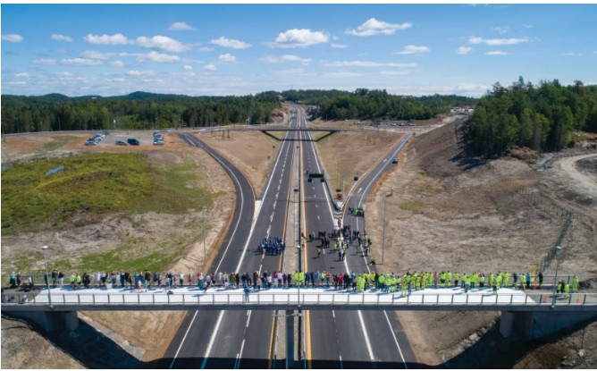
Figure 3. Opening of a new segment of E18 in Norway, included workers of the project (2021). Source: Nye Veier.
